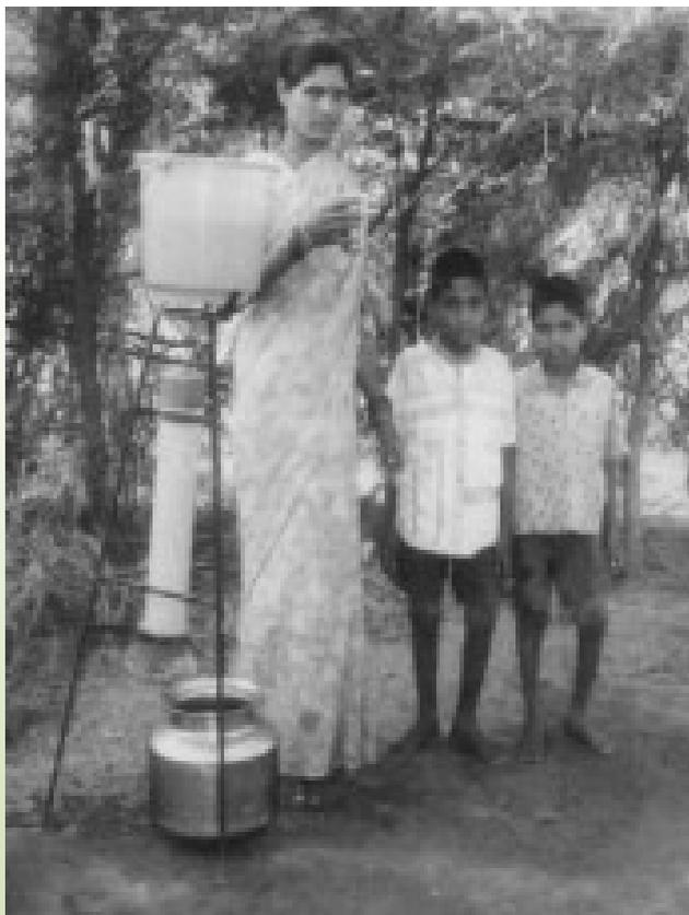
**FIGURE 1.** The utilised bone char filter.
